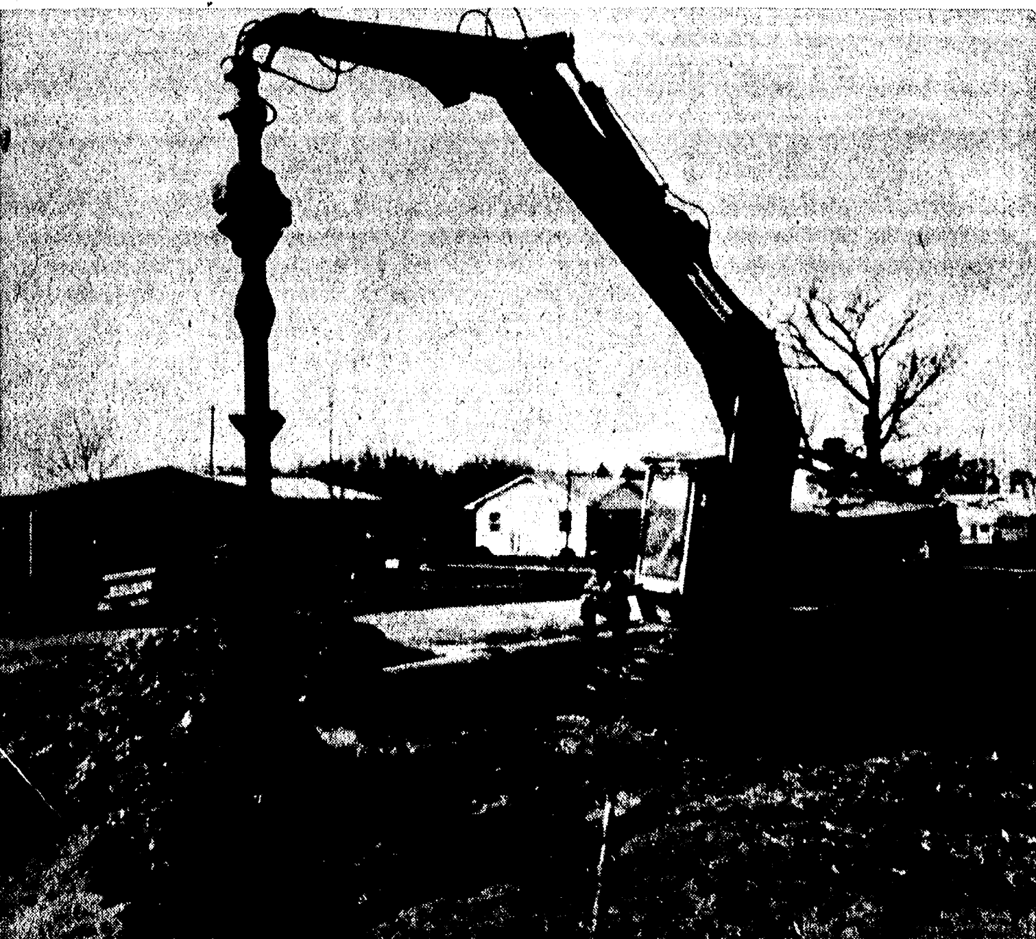
GROUND WATER has become a problem in the construction of an extension of the existing sewer that runs some 700 ft. north of Mayer Dr., and serves residents along that route. At present, workers have returned to the project from other
